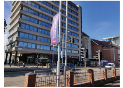
Newly installed crossing close to Trent Bridge stadium on the busy A6520 Radcliffe Road
